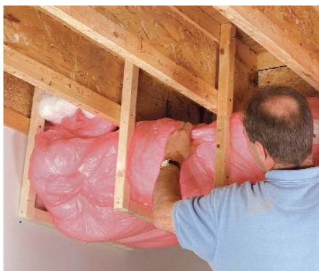
Stuff the airspace with thermal insulation. Fill the airspace around the duct with good-quality fiberglass insulation. Higher R-values dampen noise more effectively.
